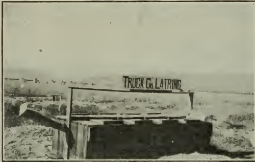
FIG. 78.—Extemporized latrine box.
